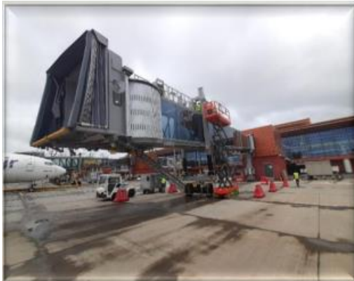
Passenger Boarding Bridge
