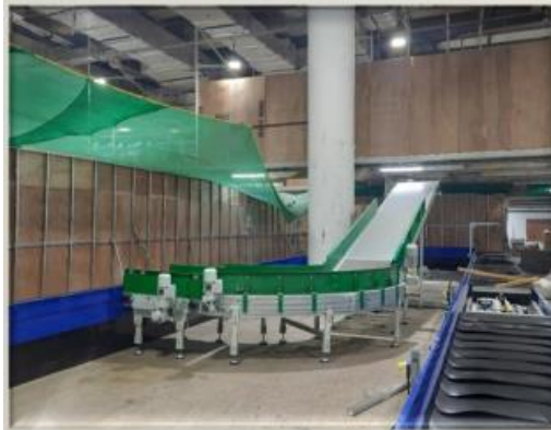
Baggage Handling Works
