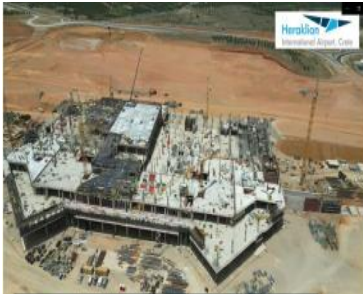
Terminal Building Structural Concreting works
