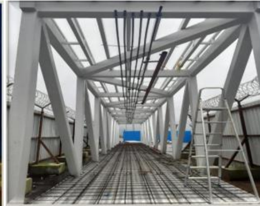
Fixed Link Bridge
